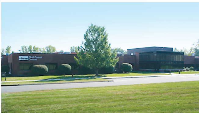
Fluid Control Division Headquarters, New Britain, CT.
