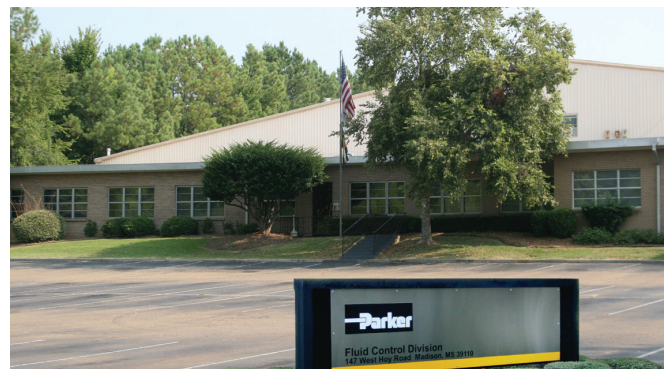
Fluid Control Division Facility, Madison, MS.
